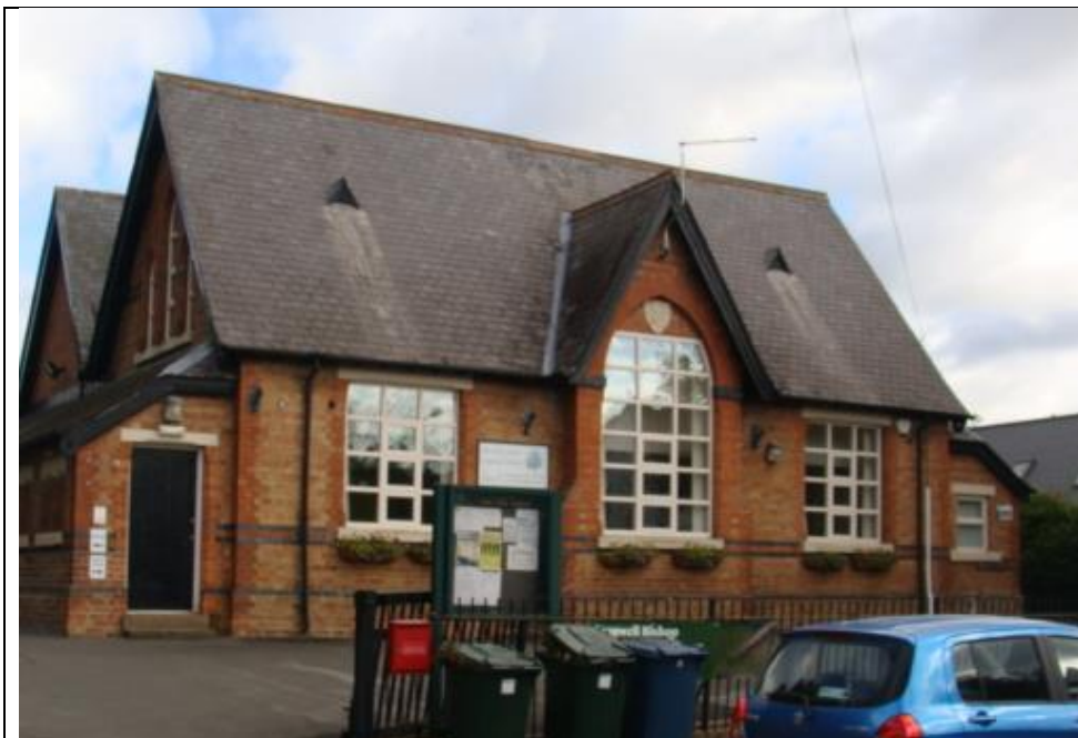
The former village school was built in 1878 and has the typical 'gothic' design influences of civic buildings of the high Victorian period.
