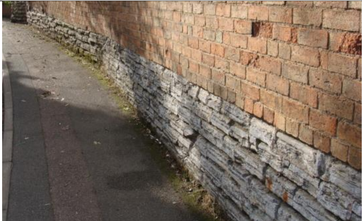
A widespread feature seen around the village are boundary walls featuring stone plinths or footings, commonly either in blue lias or grey marl. Whilst walls entirely built of stone do exist they are less common.
